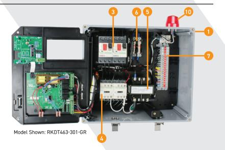
The RK Series™ Three Phase Duplex 4-20 mA continuous level sensing panel is designed to control two 208/230/460 VAC three phase pumps in water and sewage installations. The protective inner door features panel operating status indicators, LCD display, control buttons and provides access to the pump motor protection switches. The controller provides for alternation of the pumps for even usage. Panel is designed for 4-20mA input and 2-float backup control.
